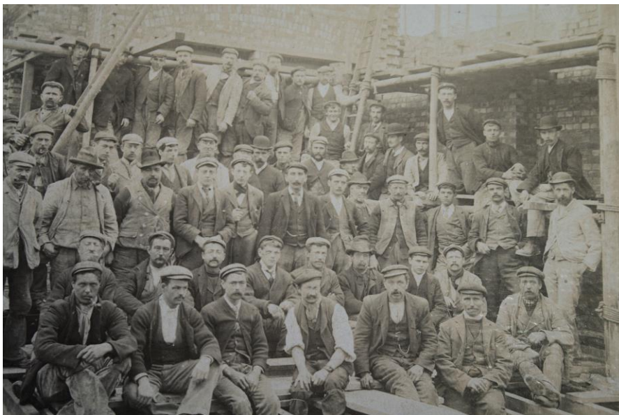
John Jarvis builders at the Opera House. c1901
